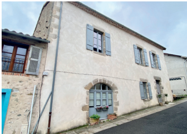
It's hard to believe that the house had broken windows and a tree growing out of the attic
